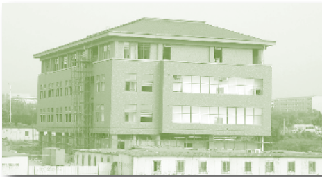
Construction of the new SGIV building is now complete
